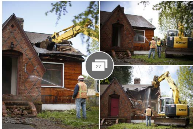
Gallery: Asbestos removal in North Portland
